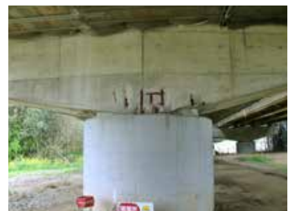
Atmospheric carbonation induced corrosion
