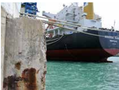
Chloride induced corrosion from sea water or de-icing salts
