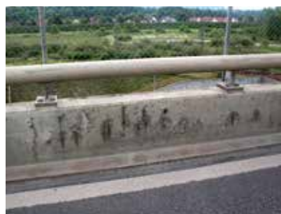
Chloride induced corrosion from sea water or de-icing salts
