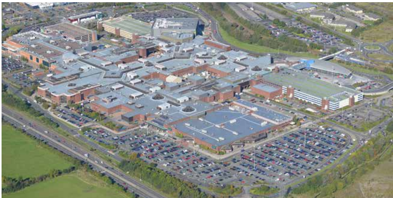
Shopping center MetroCentre (20,000 m 2 ), Gateshead, UK
