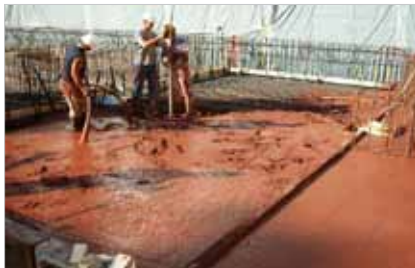
Fig. 8.16.1: The floor, walls and ceiling of this medical building were constructed with heavyweight concrete using hematite metallic aggregates to ensure full and secure radiation protection.
