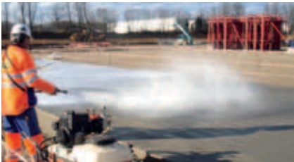
Fig. 8.10.2: Immediate coverage or curing of concrete surfaces exposed to the elements is the most crucial step for protection of such surfaces.
